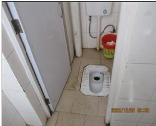
Photo of the sanitary facilities Toilet.JPG
